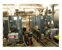
Three new energy efficient replacement boilers were installed at Westford Academy and Nabnasset Elementary Schools. Supporting calculations determined highest energy use and heat gain/loss, and were used to design and balance efficiency for the 2.5 MBH and 4.6 MBH gas boilers over the entire life cycle. Use of integrated electronic engineering, metallurgy considerations, and energy monitoring can meet or exceed planned energy demands for the years ahead.
